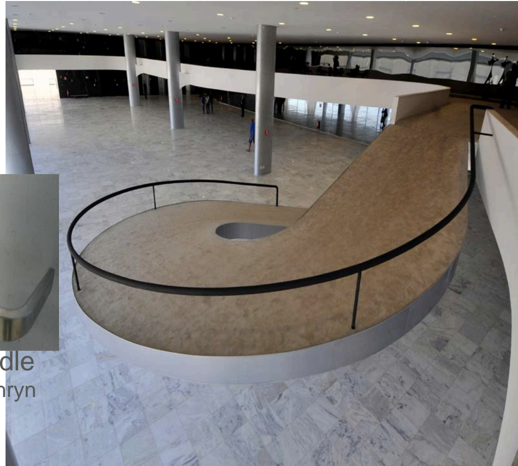
Pedestrian ramp (Photo: Limongi)
